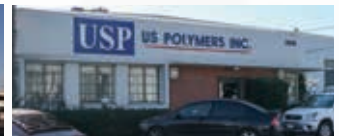
USP Extrusion Facility Commerce, California
